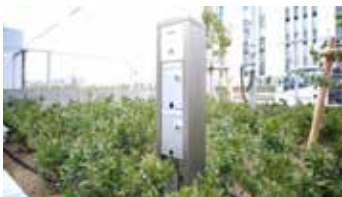
Rainwater tank capable of storing 820L
