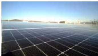
Solar panels for 78 hours of emergency power generation
