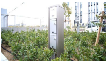
Rainwater tank capable of storing 820L
